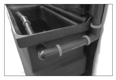
Step 34. Connect the T-full flow connector in the middle of the water tank, pointing the T downwards
